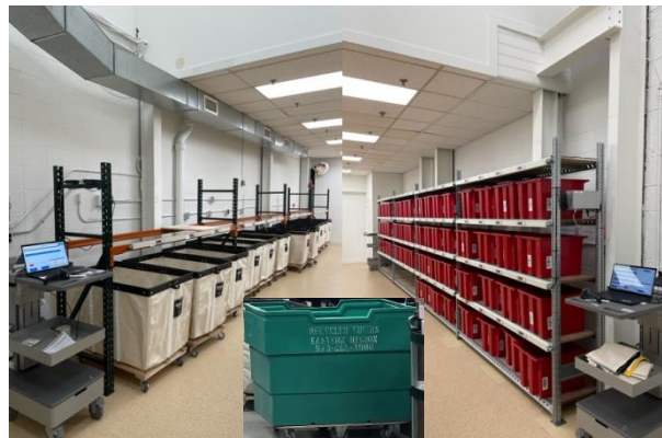
Installation of automatic return/sorting system (Put wall) completed (September FY2022)
