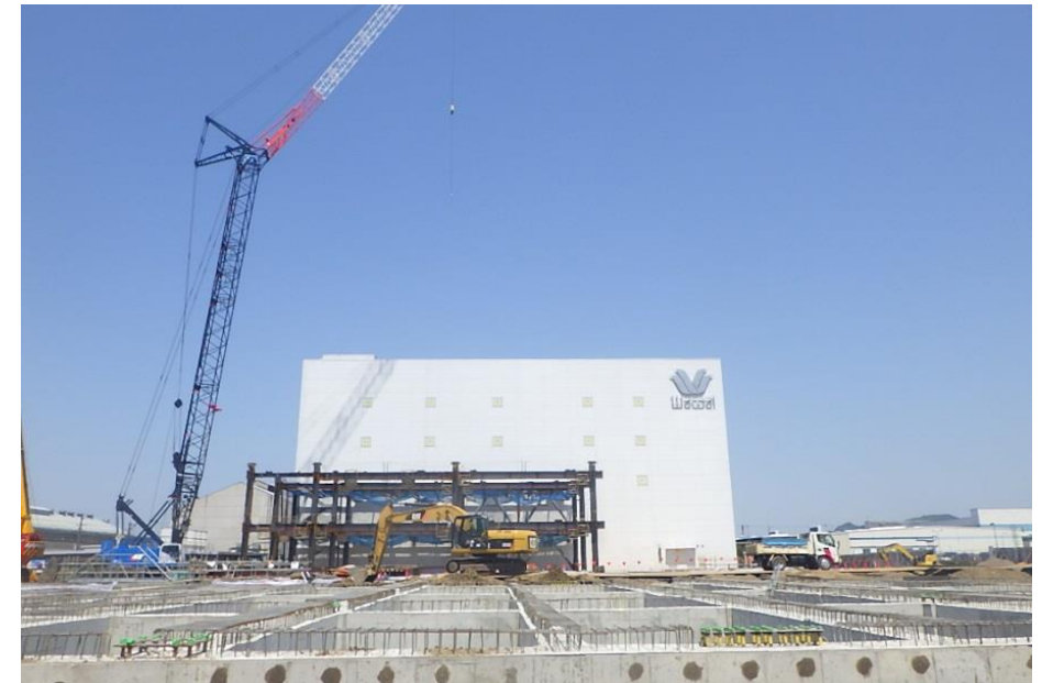
State of expansion work
